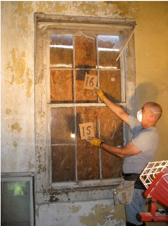
*Window "A" from interior, north elevation, showing damaged and missing muntins in both sash which will be recreated.*
